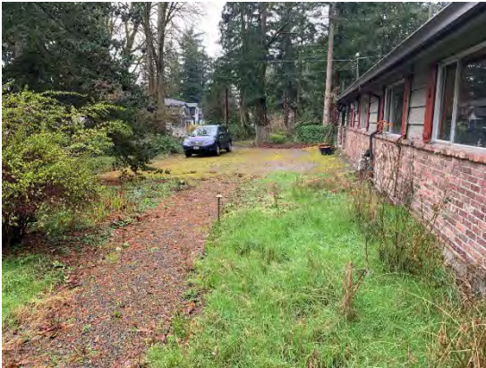
Plate 1: Existing building (south side), looking west
